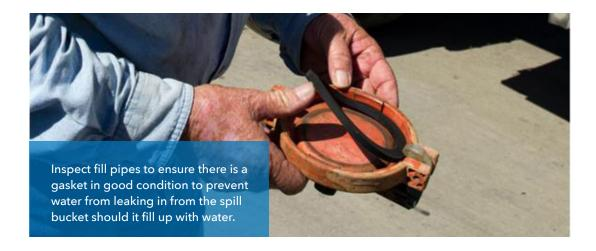
5 Inspect spill bucket lids for damaged or missing gaskets. Not all lids come with rubber gaskets, but when they do, they can help keep water out of spill buckets.
