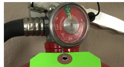
Good Needle located in Green section in operable position
