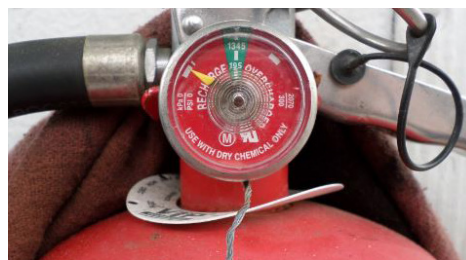
Deficiency Fire Extinguisher needing recharged.
